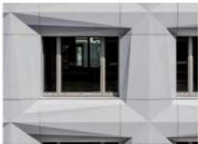
The Shift office complex in Paris by Axel Schoenert Architectes is fitted with Exteriors panels by Corian. They are based on the Corian Solid Surface in Glacier White. The architects wanted to create a plastic, three-dimen-
