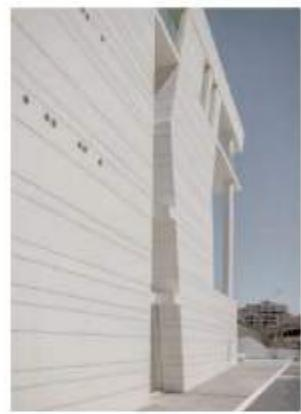
When converting the former Zedda Piras distillery in downtown Cagliari, Sicily, into a residential and commercial building, the Fadda Studio in Cagliari opted for large-format ceramic panels with minimal thickness from Laminam. The ceramic panels used were the Bianco-Assoluto tiles from the Collection series. The 5 mm-thick and 1000 x 3000 mm-large panels were cut into various sizes to completely cover the acute-angled building.
