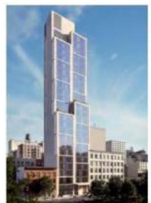
For the facade of a 25-storey commercial residential high-rise building in Manhattan, architecture firm Built from New York chose Neolith panels. In order to keep maintenance costs as low as possible, the panels were treated with a Pureti water-based photocatalytic solution that makes the material hydrophilic and self-cleaning. 2000 m<sup>2</sup> of the Pureti-treated Jura Limestone from Neolith cover the facade and frame the 3-storey glass surfaces on the front of the building.
